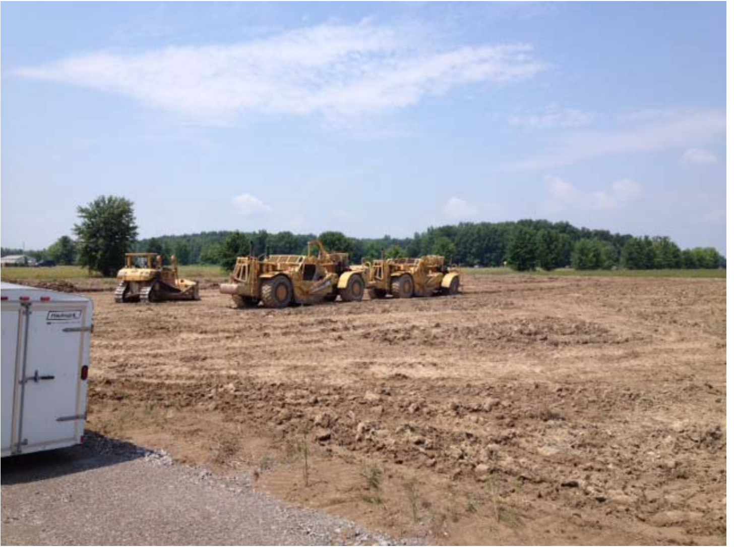
Ongoing Topsoil Stripping Being Completed By Nelson Stark
