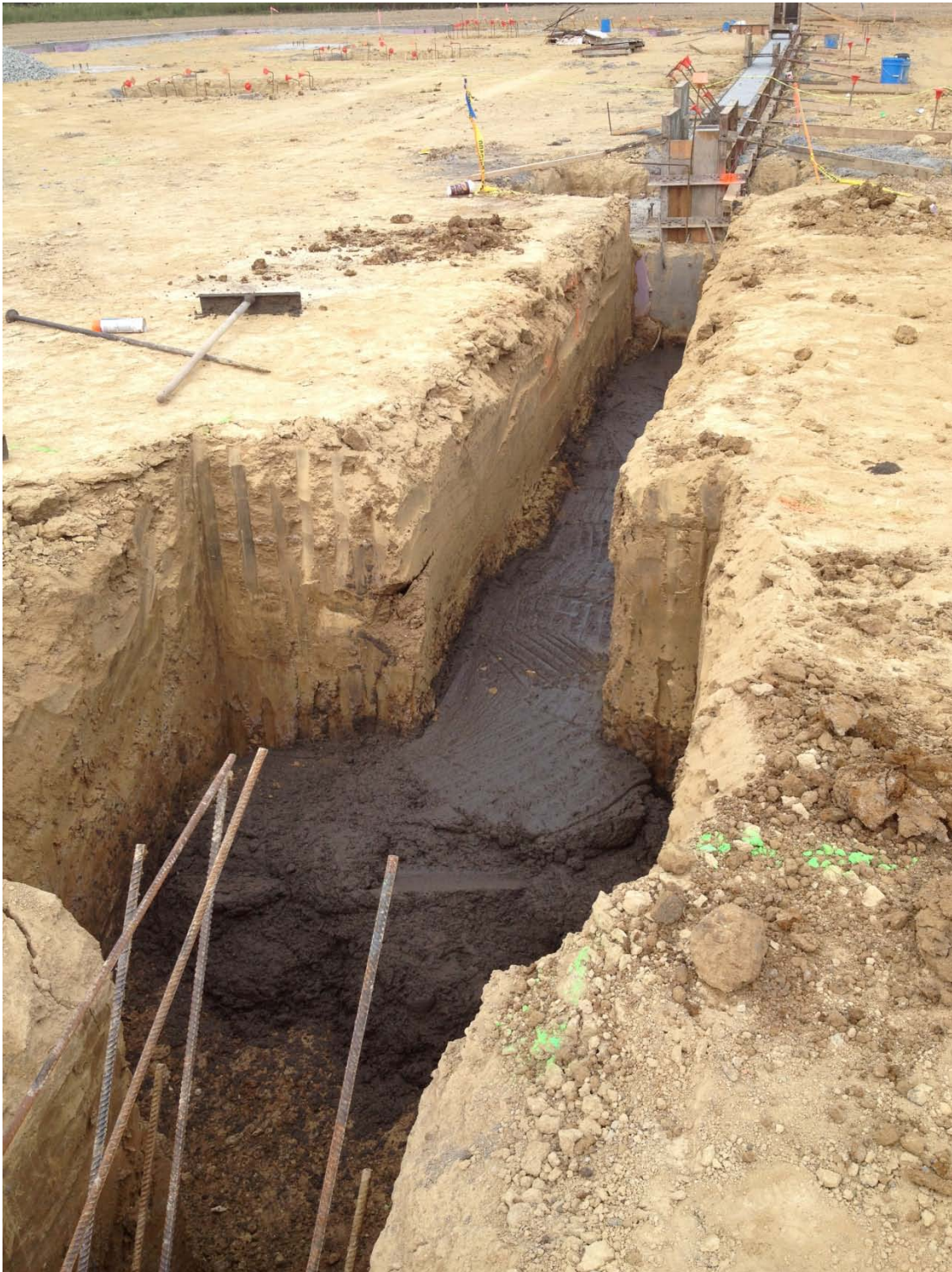
Leancrete Poured at Last Footing Location
