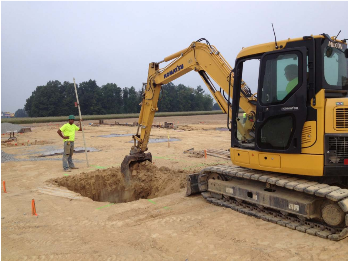
Digging the Elevator Pit
