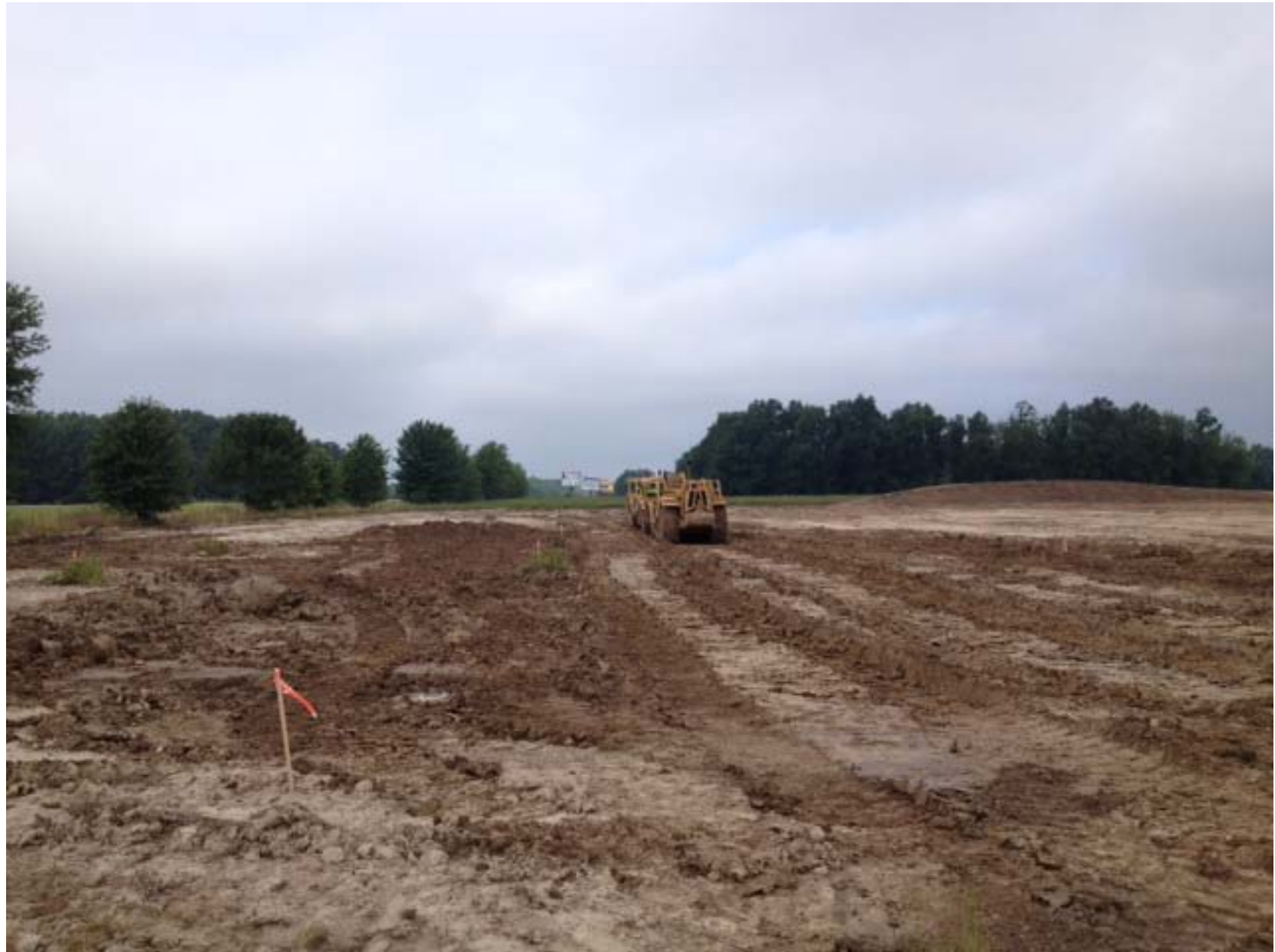
Nelson Stark Beginning Excavation of the Pond
