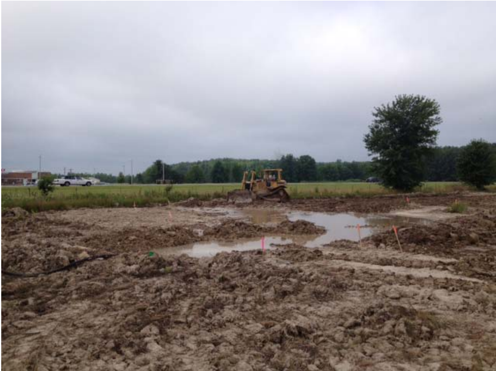
Removing Site Water
