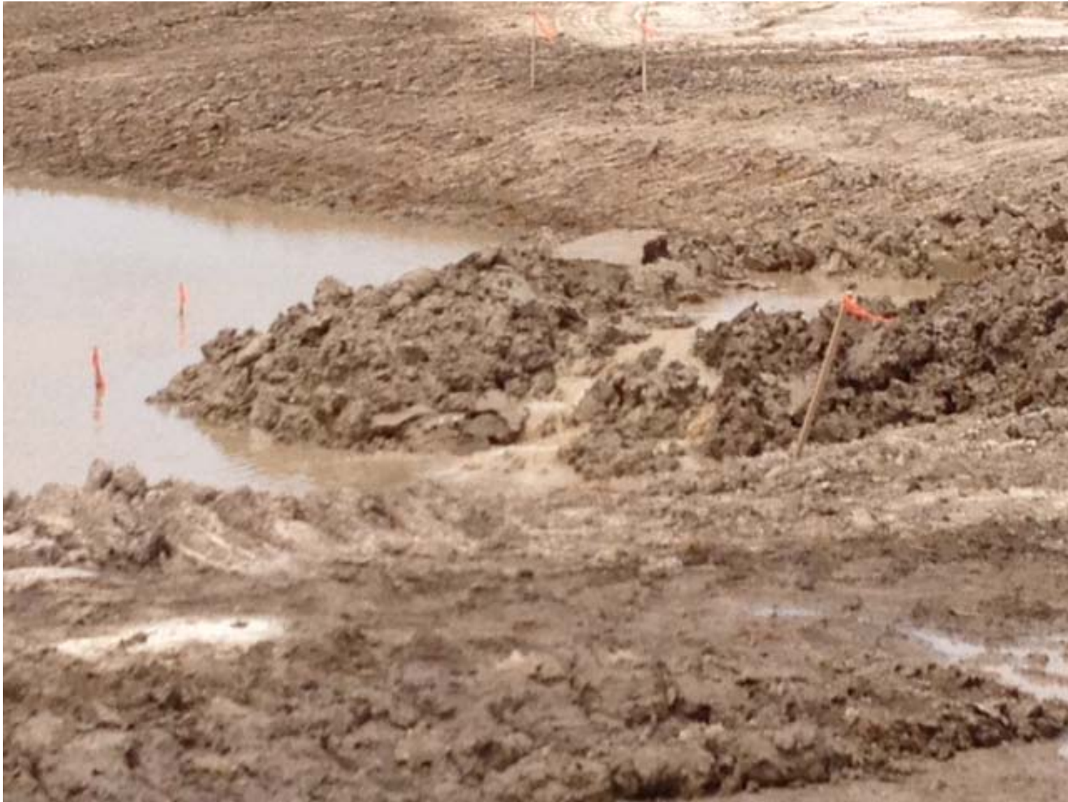
Site Dewatering Taking Place
