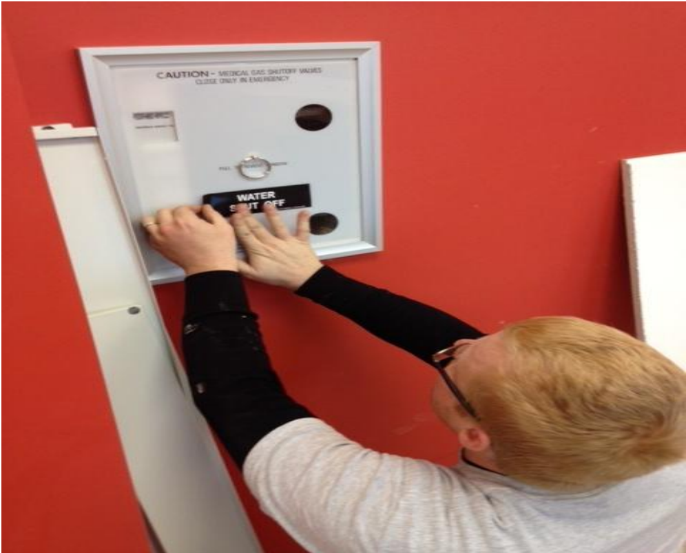
Applying labels on shut-off valves
