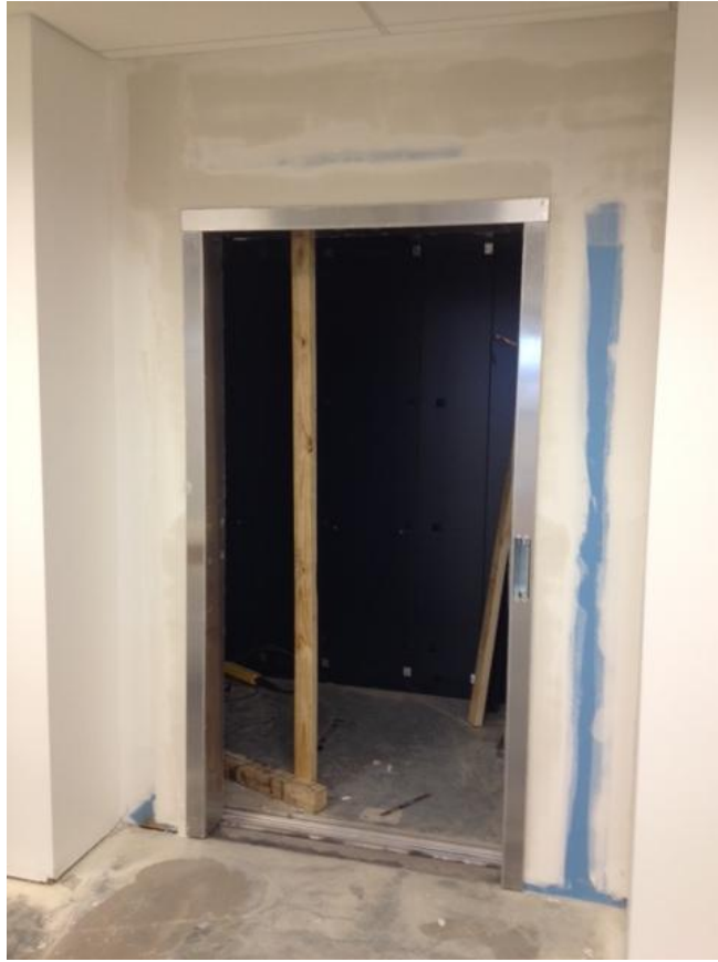
Finishing drywall at elevator doors 2 nd floor
