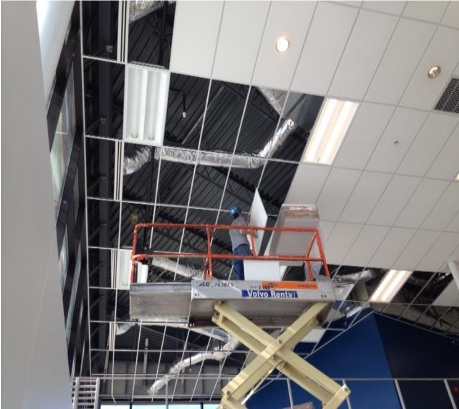
Continuing lobby ceilings
