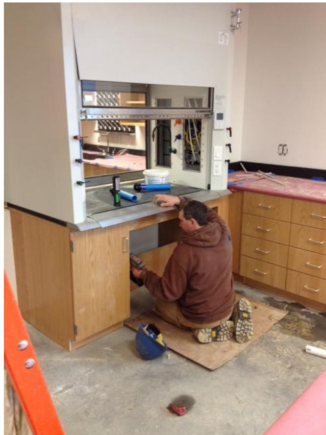
Finishing last fume hood utilities
