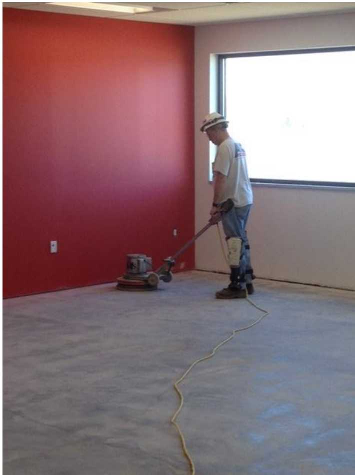
Sanding floors for carpet in classroom 2 nd floor
