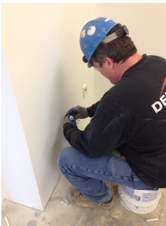
Installing 2 nd floor wall outlets
