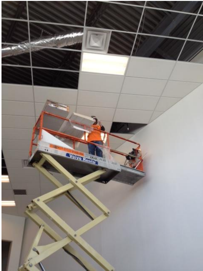
Installing lobby ceiling tile
