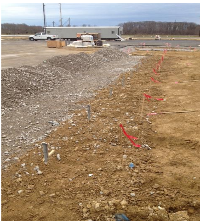
Sidewalk light bollard electric roughed in
