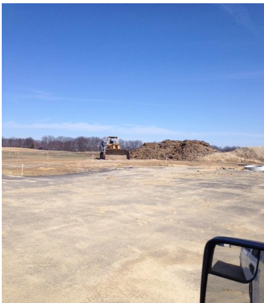
Starting the topsoil stripping at new maintenance building
