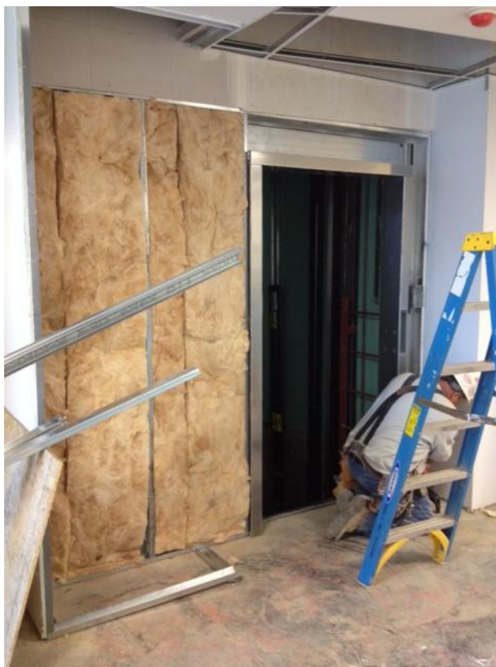
Finishing the drywall at the elevator openings
