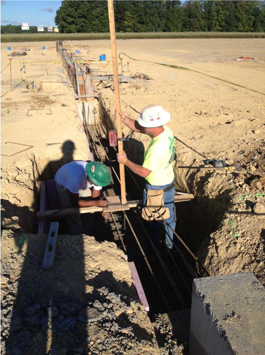
Installing Footing Rebar in the Last Location
