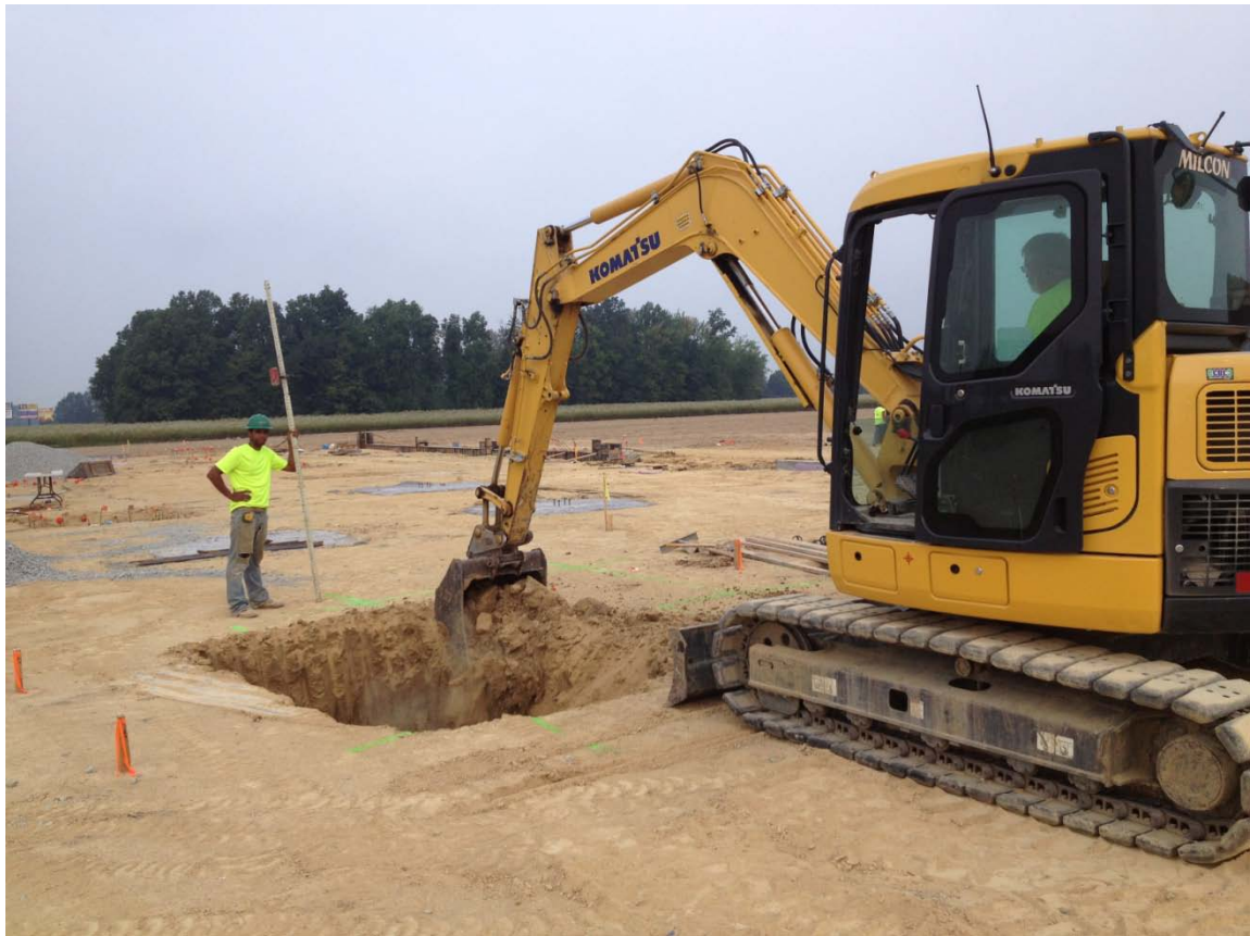
Digging the Elevator Pit
