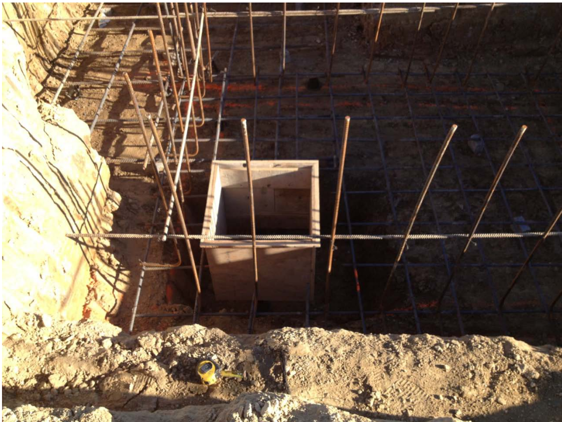
Rebar and Sump Pit Forms Installed for the Elevator Pit
