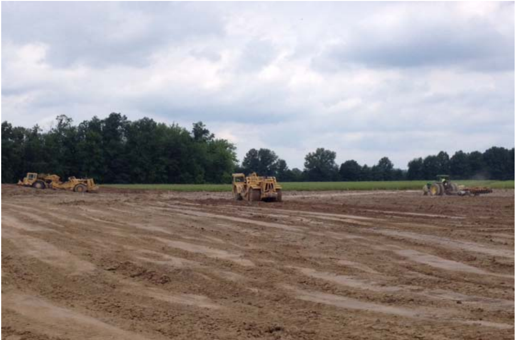
Nelson Stark Completing Topsoil Removal
