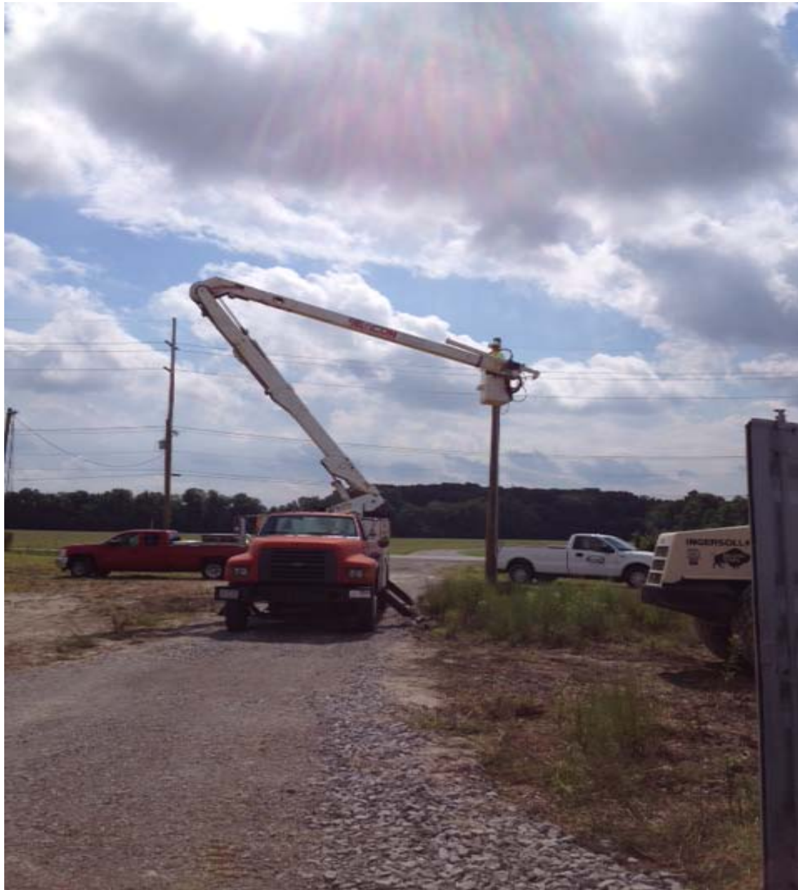
Beacon Electric Setting the Pole for Temporary Power
