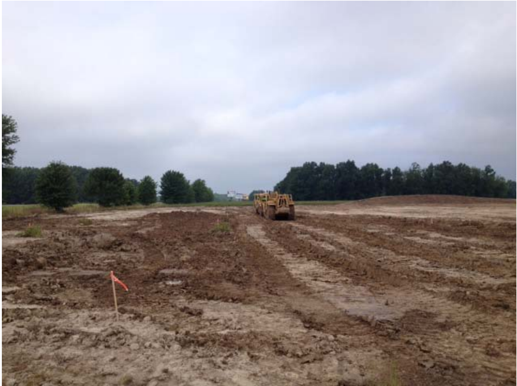
Nelson Stark Beginning Excavation of the Pond
