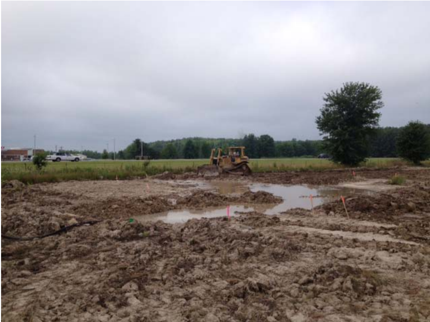
Removing Site Water
