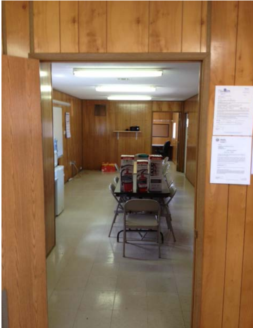
Site Office Temporary Power Complete
