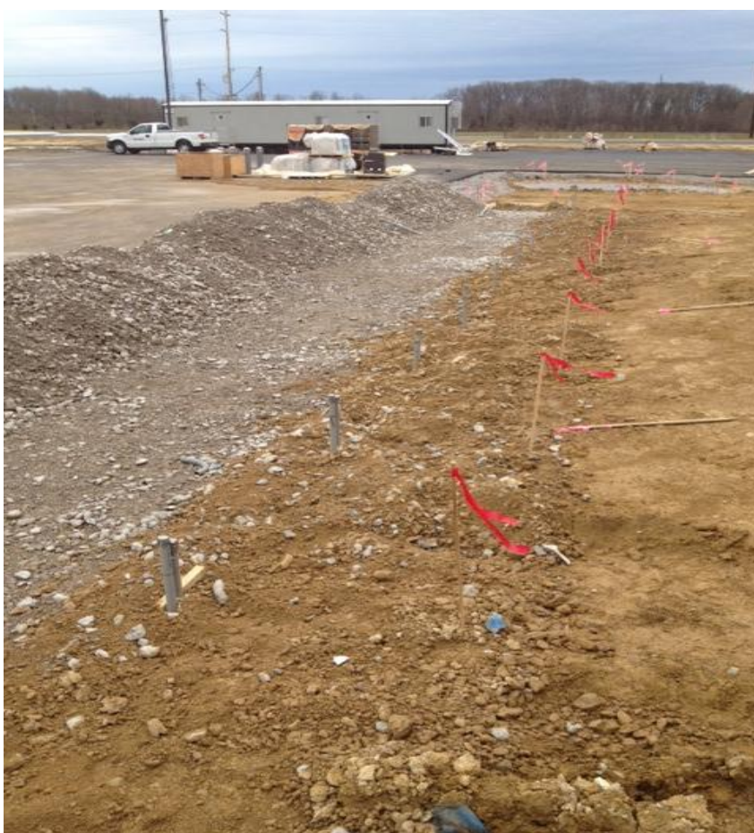
Sidewalk light bollard electric roughed in
