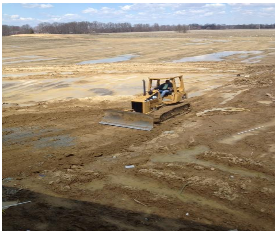
Re-grading around north side of building
