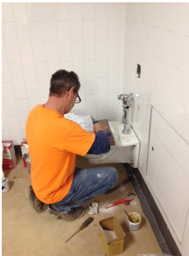
Installing flush valves on restroom fixtures
