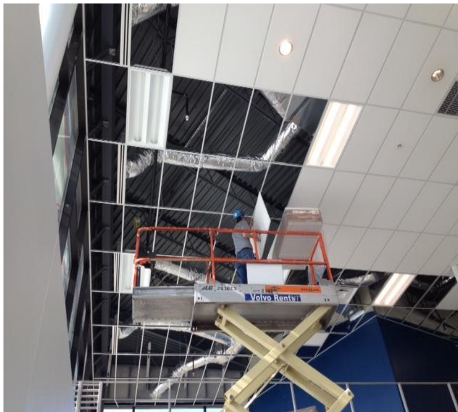
Continuing lobby ceilings
