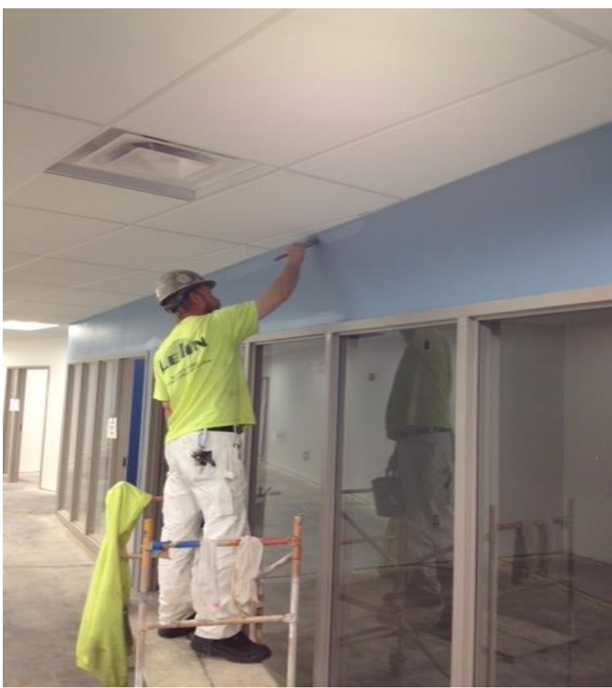
Applying final coat paint in 2 nd floor corridor
