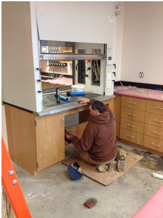
Finishing last fume hood utilities
