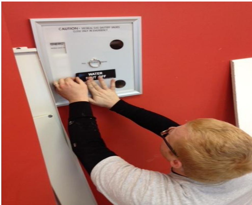
Applying labels on shut-off valves
