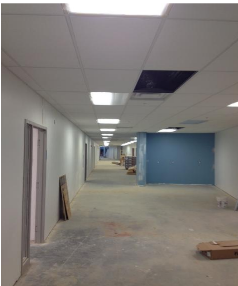
1 st floor corridor ceilings completed
