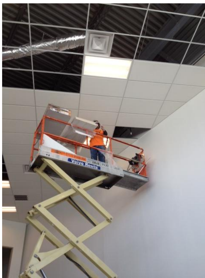
Installing lobby ceiling tile
