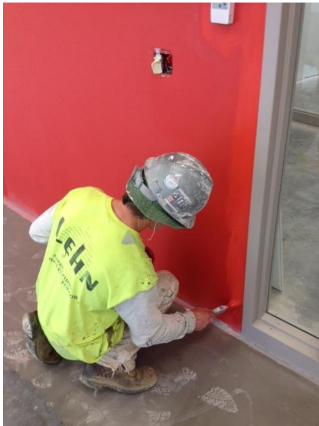
Cutting in for final coat paint on accent walls 2 nd floor
