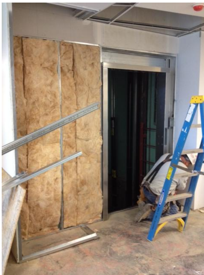
Finishing the drywall at the elevator openings
