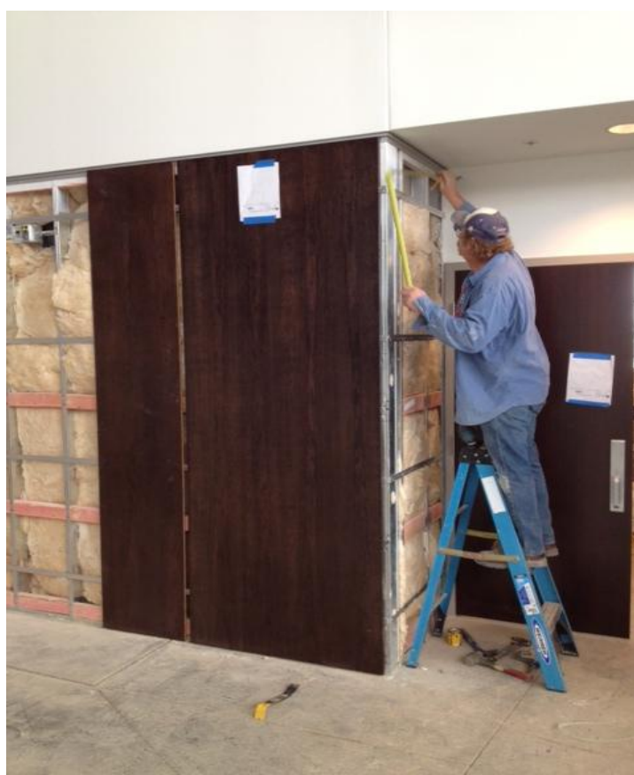
Installing cherry wall panels
