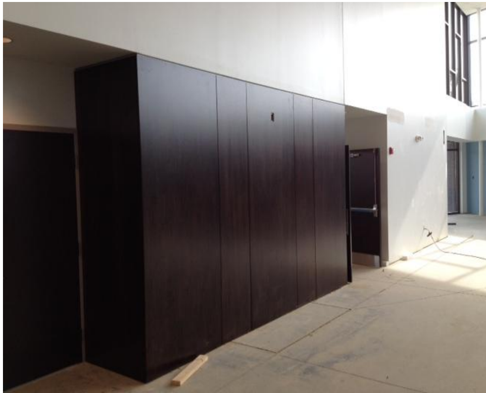
Cherry wall panels installed
