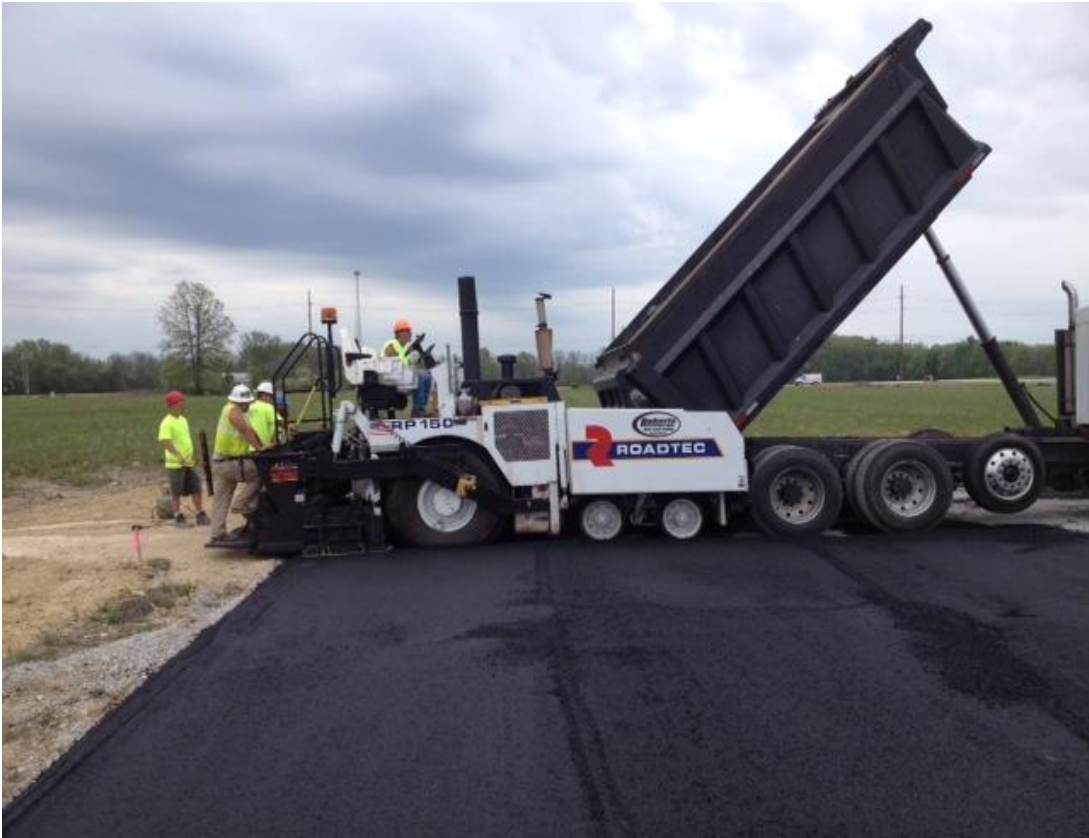
Paving the maintenance road
