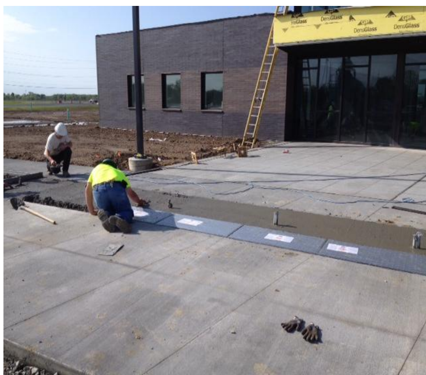
Installing the ADA mats at drop off area
