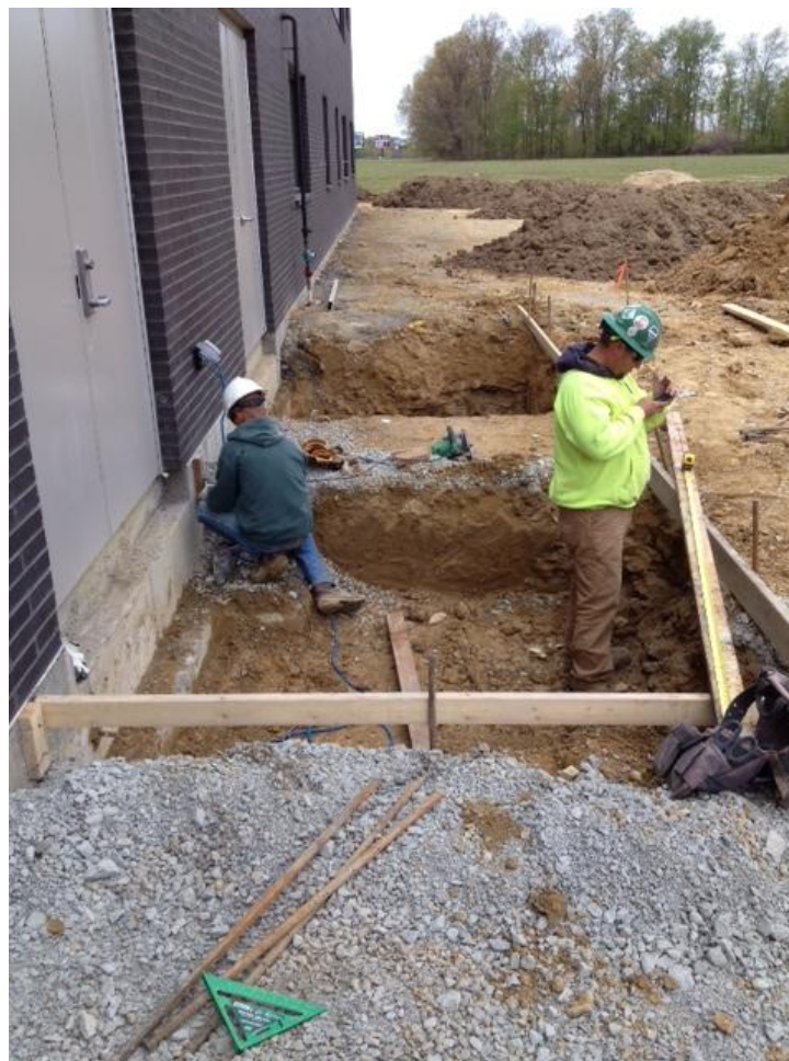
Prepping for frost slabs at exit doors
