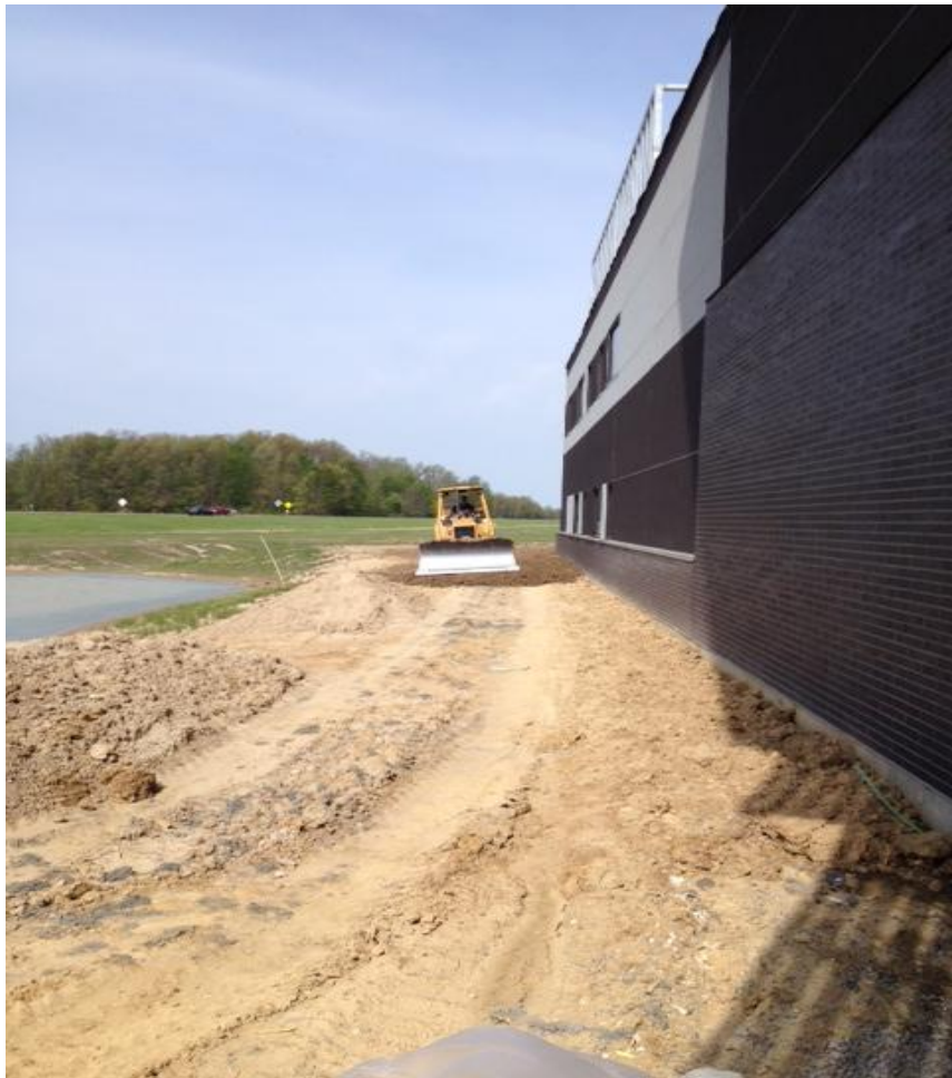
Installing topsoil around pond area
