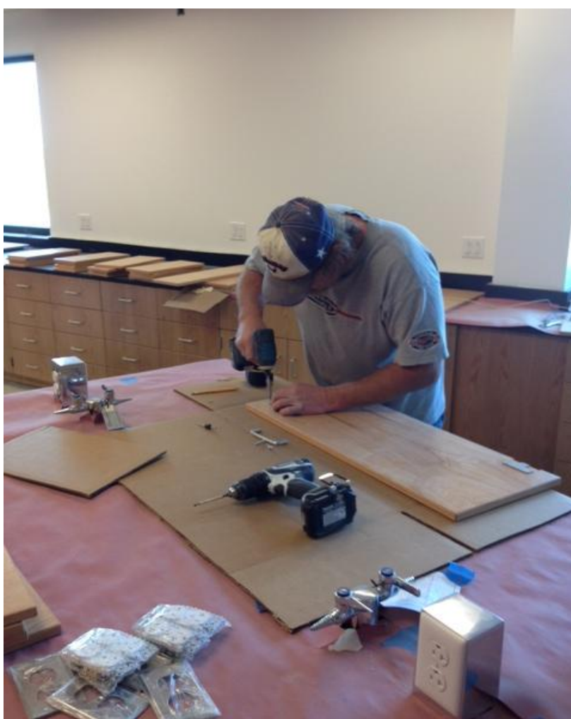
Replacing science lab doors
